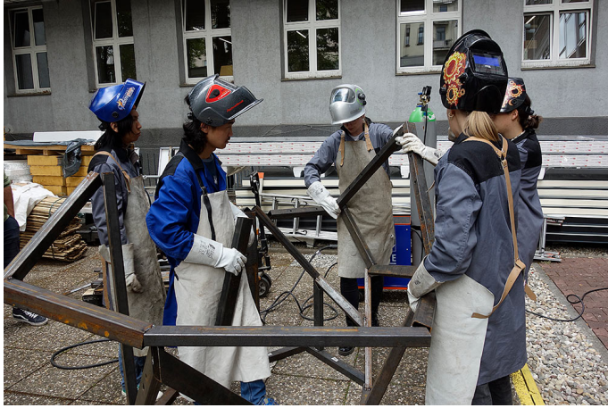
Welding in the courtyard
